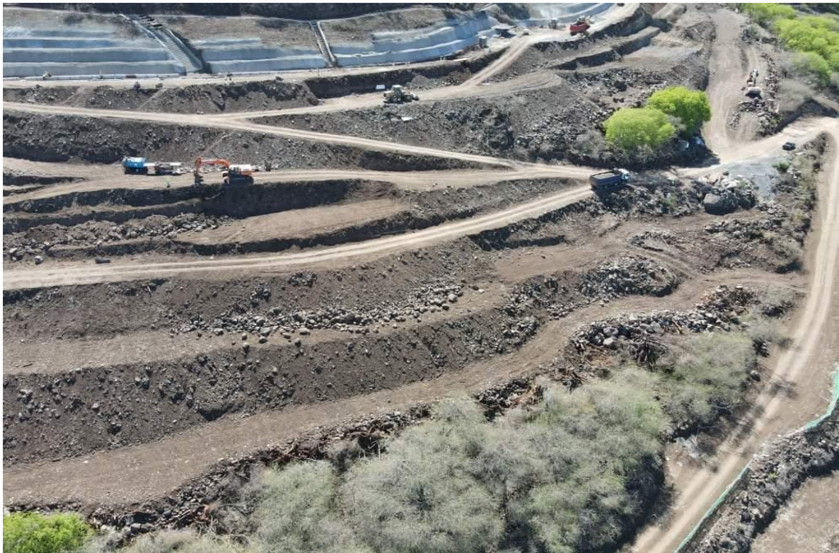
Photo 2 – The mountain side is being terraced at slopes between 33-40% grades that far exceed the 20% grade permissible construction limit under the country's Planning Policy Guidance (PPG) on Development on Sloping Sites and Landslide Hazard Areas.
